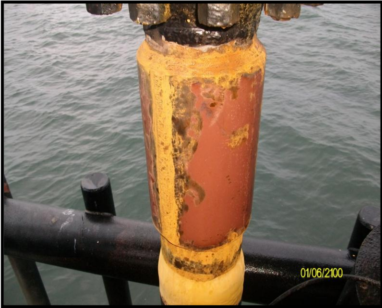
Before Picture (previous splash zone protection product cut back)
