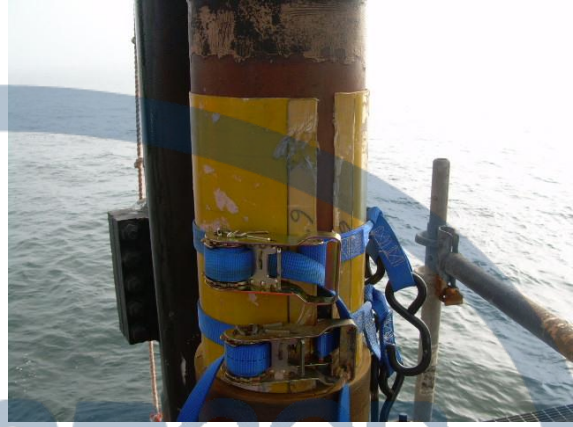
Clock Spring Single Wrap Molding Process
