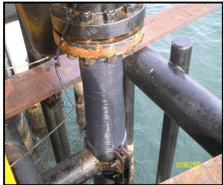
4" Riser after RiserWrap Installation.
