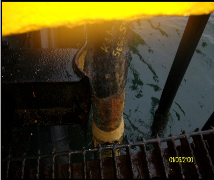
Before Picture of 4" Riser with previous splash zone protection product cut back
