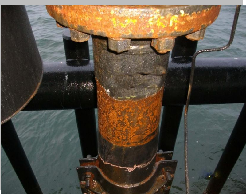
Before Picture of 4" Riser with previous splash zone protection product cut back
