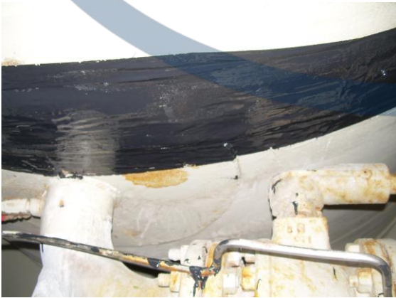
Close-Up of Leak Repair Area with RiserWrap Installation
