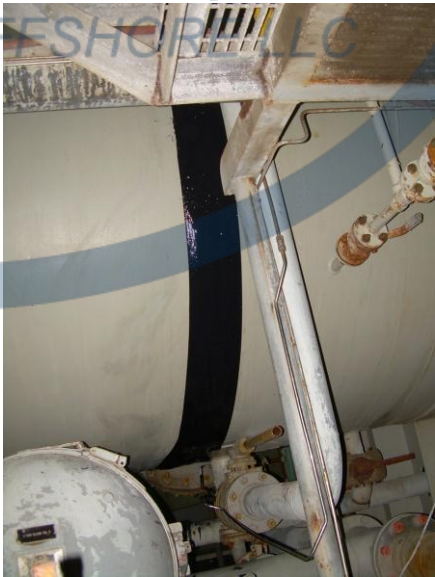
Overview of Completed Installation
