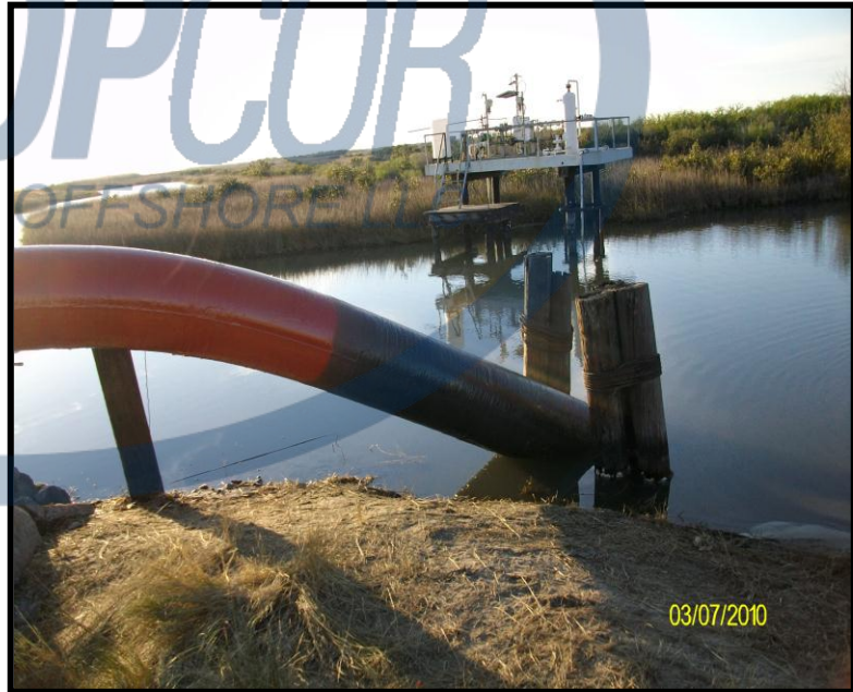
Completed RiserClad-RiserWrap Installation
